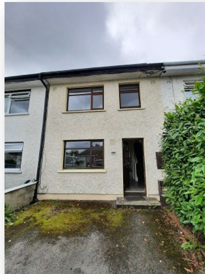
Figure 1 – Ater – Refurbishment, Deep Retrofit
