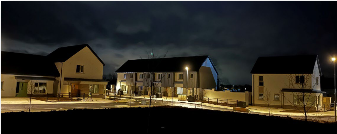
Completed Development at Coill Dubh
